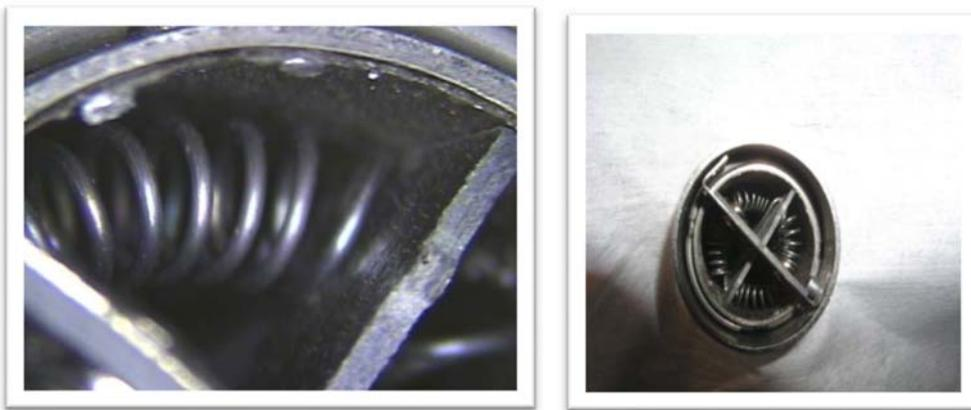
**Figure 8. APR Open Coil Convection Heaters**
